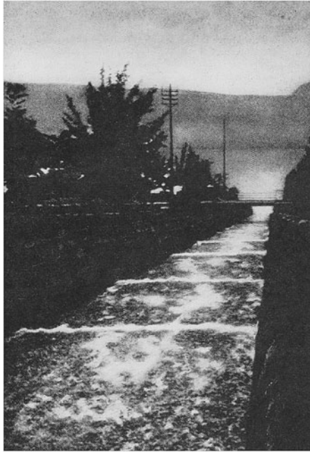
Fig. 6.15 Roll waves, looking downstream (The Grünbach, Switzerland). From Stoker (1957).
