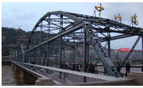
The Lanzhou Zhongshan Bridge
